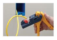
Ensure jack is completely and securely inserted in jack holder bed with IDC slots facing the blades.
